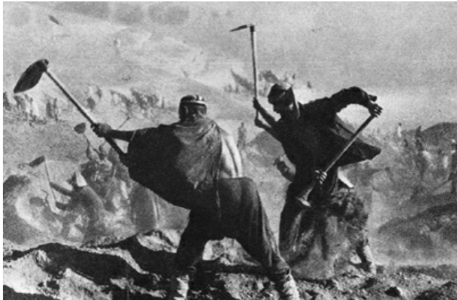
11a Digging the Fergana Canal
