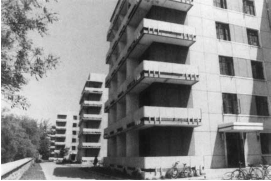
FIGURE 8.2. The master's student dormitories at Beijing University. (Photograph by the author.)
