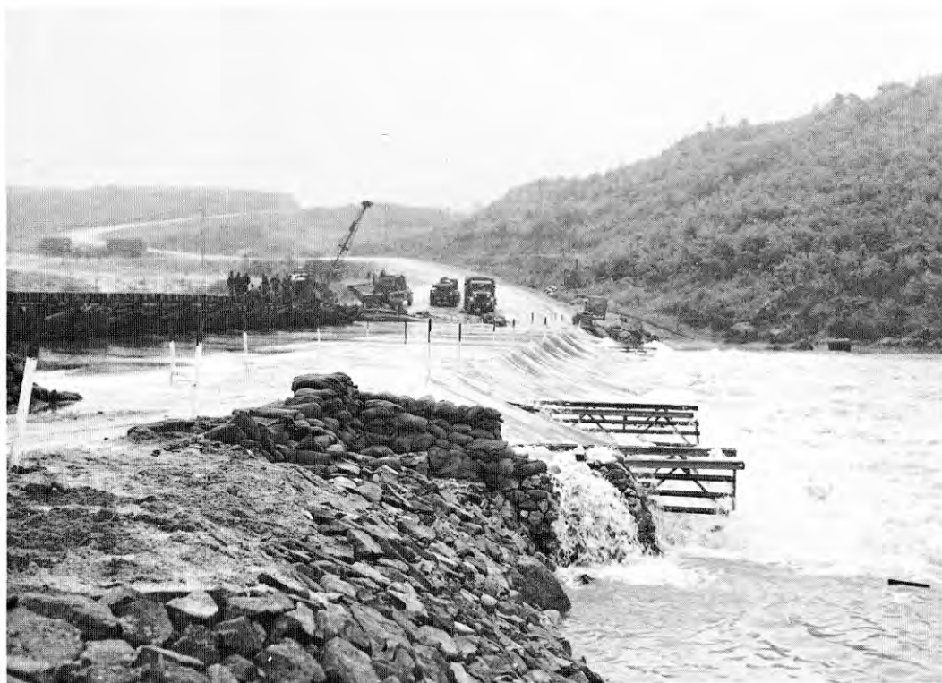
FLOODED BRIDGE CROSSING ON THE MAIN SUPPLY ROUTE, CH'ORWON VALLEY
